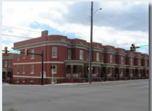
Minvilla Manor (formerly the 5th Ave. Motel) which is on the National Historic Register.
