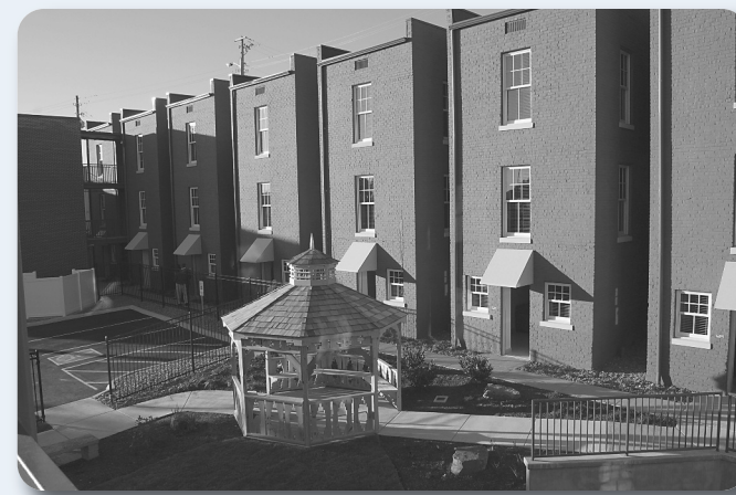
Garden level apartments
